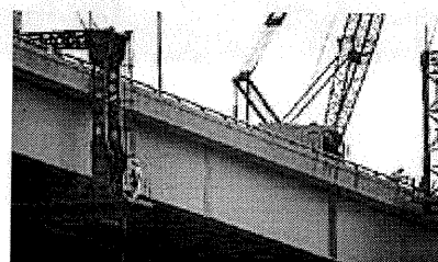
Photo/Jack Orton Department of Transportation workers prepare to inspect the underside of the Hoan Bridge's southbound lanes Thursday. A hairline crack turned up in one of three girders supporting those lanes - near where a section of northbound lanes had to be demolished after girders failed.
