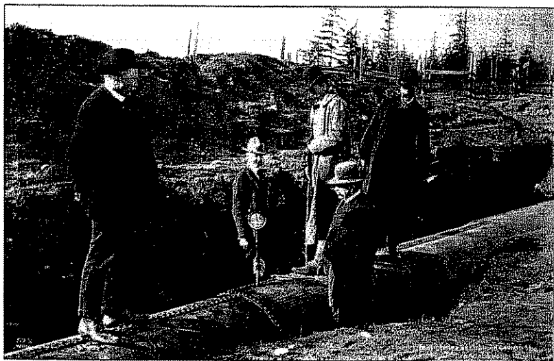
▲ Vintage. Like other cities, Seattle's water pipes and sewer system are showing their age.
