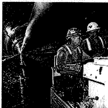
Workers Michael Robison, right, and David Splendiani tour the Nancy Creek Tunnel project in Atlanta.
