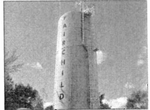
Water Storage Standpipe Replacement Project
