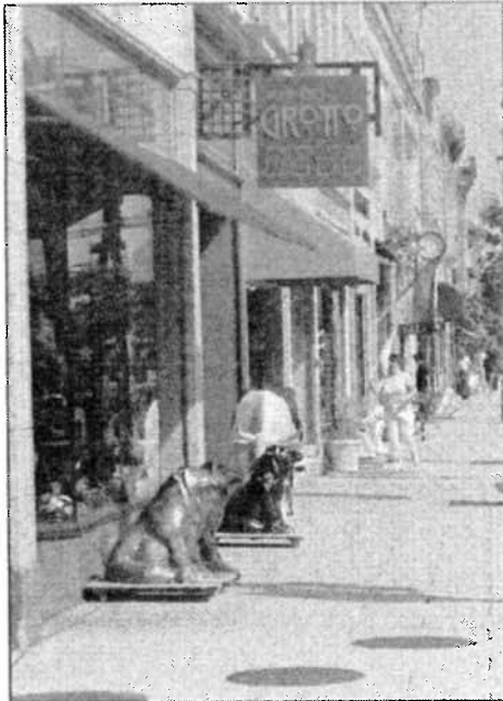
The Racine Main Street Streetscape Project features redesign and reconstruction from storefront to storefront.
