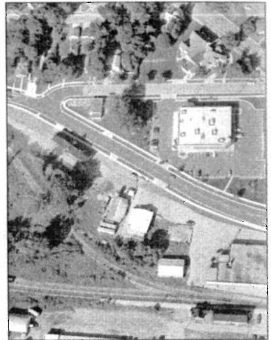
Hattie Street Brownfield Redevelopment
