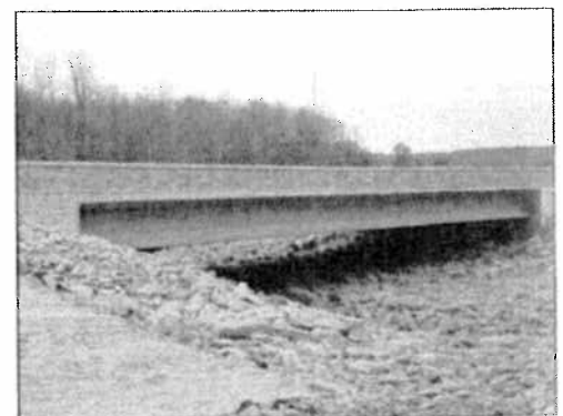
Alfred Benesch & Co.'s completed bridge project features the first bridge deck in Wisconsin reinforced with a prefabricated FRP reinforcement cage.
