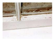
Chipping paint is deteriorated paint and must be repaired.
