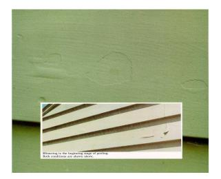
Blistering paint is deteriorated paint and must be repaired.
