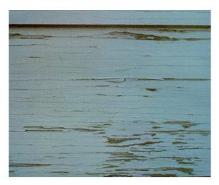
Checking paint is deteriorated paint and must be repaired when an adhesion test determines that any layer is not securely bonded. To conduct an adhesion test, firmly press a  $2'' \times 2''$  piece of masking tape to the suspect paint and rub the tape to adhere firmly. Lift up on one corner of the tape and remove the tape. If paint is evident on the tape, the paint is separating from the substrate or from underlying paint, and is not securely bonded.
