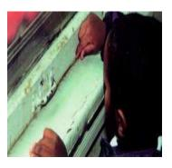
Paint affected by the mildew is deteriorated paint and must be repaired when an adhesion test determines that any layer is not securely bonded. To conduct an adhesion test, firmly press a  $2'' \ge 2''$  piece of masking tape to the suspect paint and rub the tape to adhere firmly. Lift up on one corner of the tape and remove the tape. If paint is evident on the tape, the paint is separating from the substrate or from underlying paint, and is not securely bonded.
