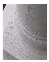
Cracking paint and cracked paint at a settlement crack is deteriorated paint and must be repaired when an adhesion test determines that any layer of paint is not securely bonded. To conduct an adhesion test, firmly press a  $2'' \ge 2''$ piece of masking tape to the suspect paint and rub the tape to adhere firmly. Lift up on one corner of the tape and remove the tape. If paint is evident on the tape, the paint is separating from the substrate or from underlying paint, and is not securely bonded.
