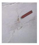
Paint that is not securely bonded is deteriorated paint and must be repaired. To conduct an adhesion test, firmly press a  $2'' \times 2''$  piece of masking tape to the suspect paint and rub the tape to adhere firmly. Lift up on one corner of the tape and remove the tape. If paint is evident on the tape, the paint is separating from the substrate or from underlying paint, and is not securely bonded.
