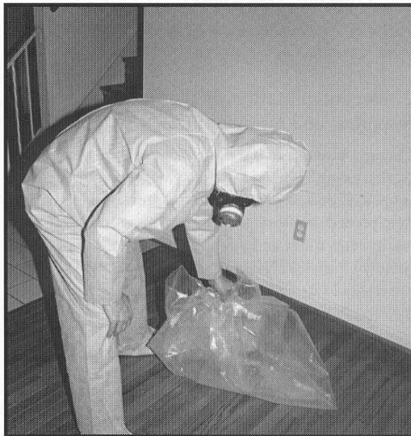
Figure 14.8b Fold Plastic Inward.
