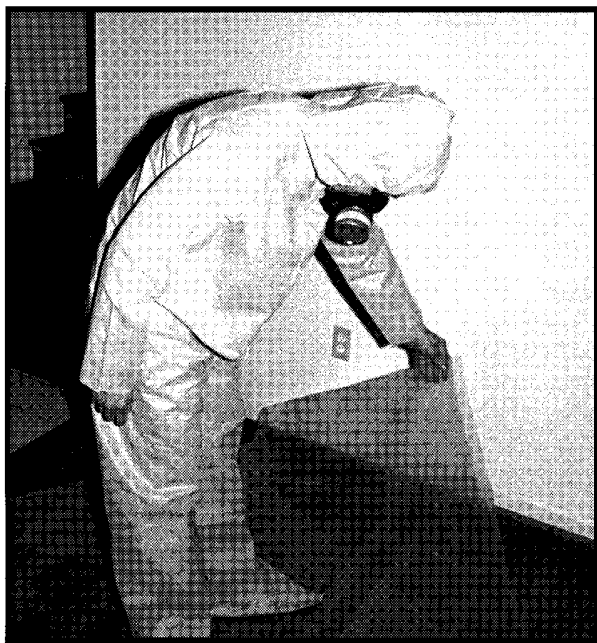
Figure 14.8a Pick Up Corners of Plastic Sheeting.
