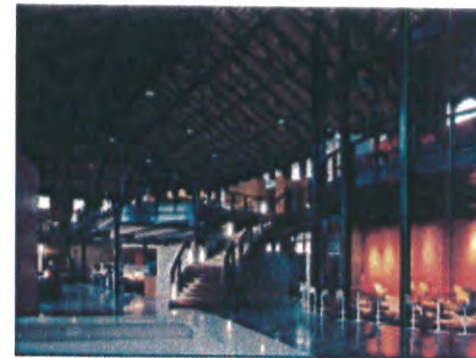
The 1902 Milwaukee Gas Light Company
