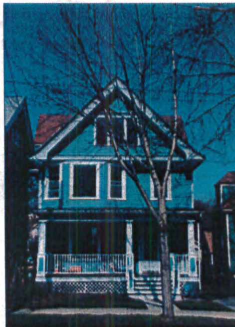
Rehabilitated home in Madison's Orton Park Historic District
