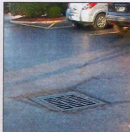
Runoff from coal-tar-sealcoated pavement goes down storm drains to receiving water bodies. The runoff contains high concentrations of PAHs and related chemicals that can harm aquatic life. 16
