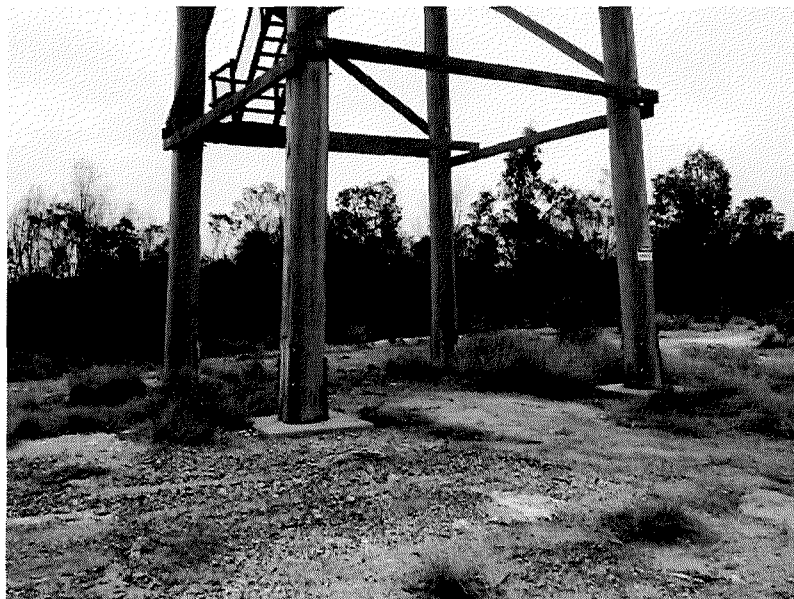
Waaje Tower and columns posted at the bottom
