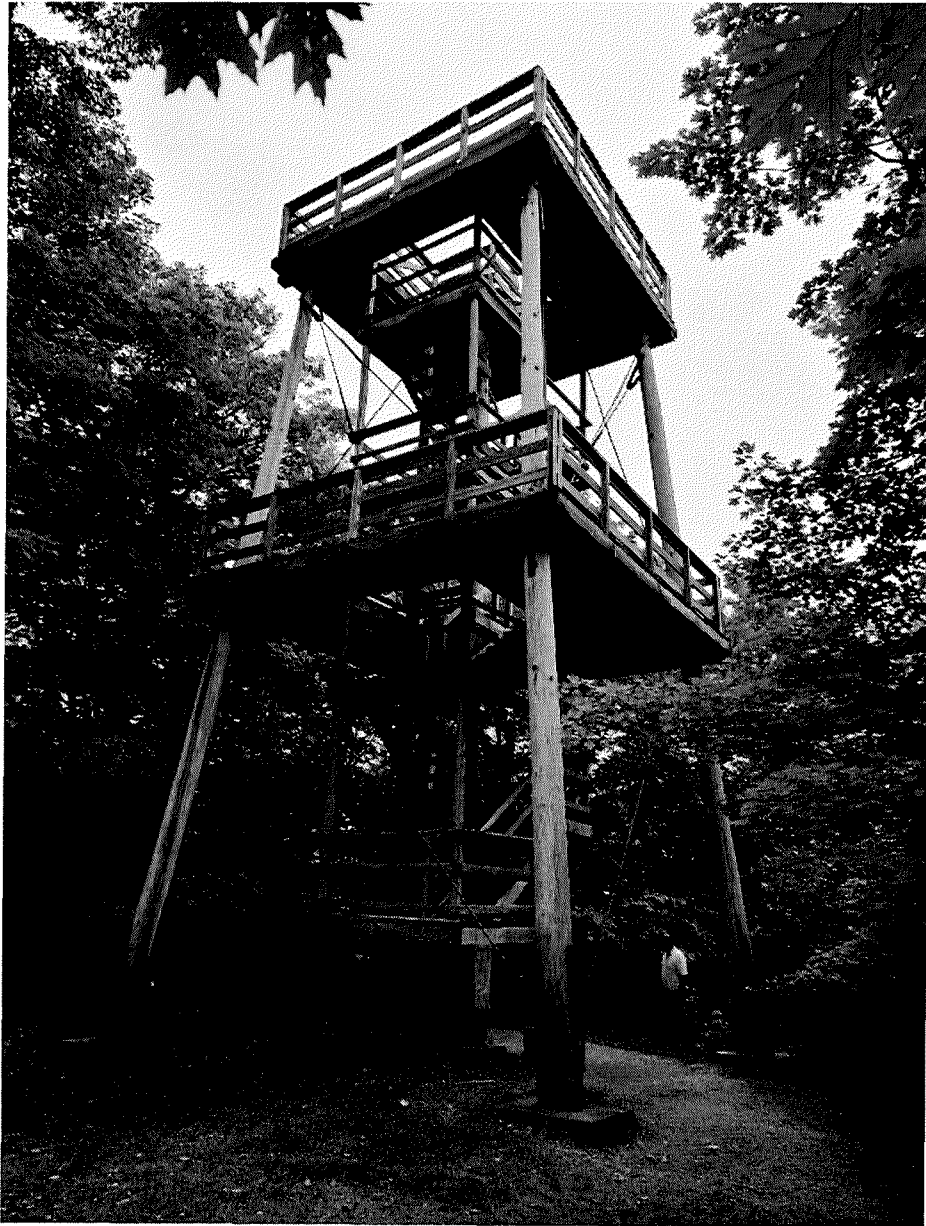
Washington Island Tower
