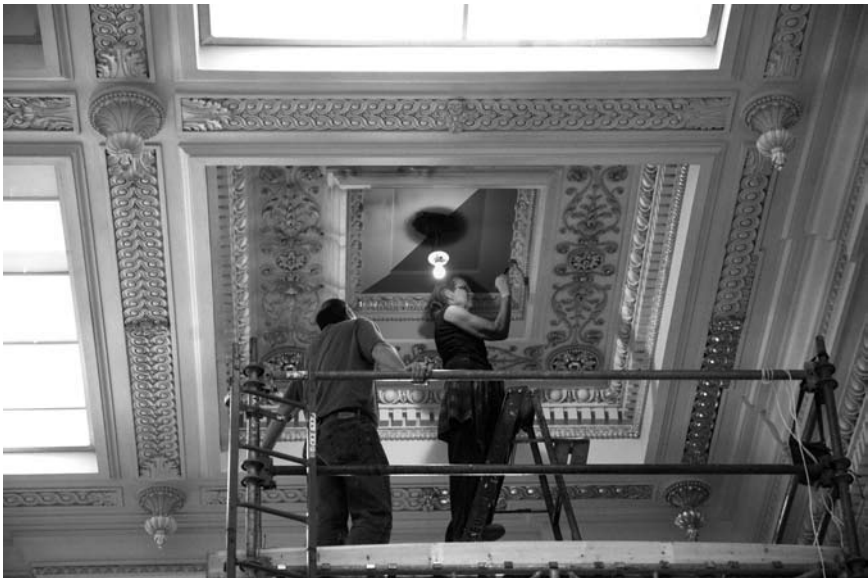
After exhaustive research, the Wisconsin Historical Society has undertaken a project to restore the grandeur of the Library Reading Room, one of the great architectural spaces in the state. When completed, the reading room will also meet the needs of modern researchers. (State Historical Society of Wisconsin)
