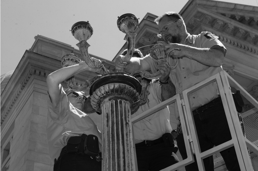
Department of Administration employees repair outdoor lighting at the State Capitol. (Greg Anderson, Legislative Photographer)
