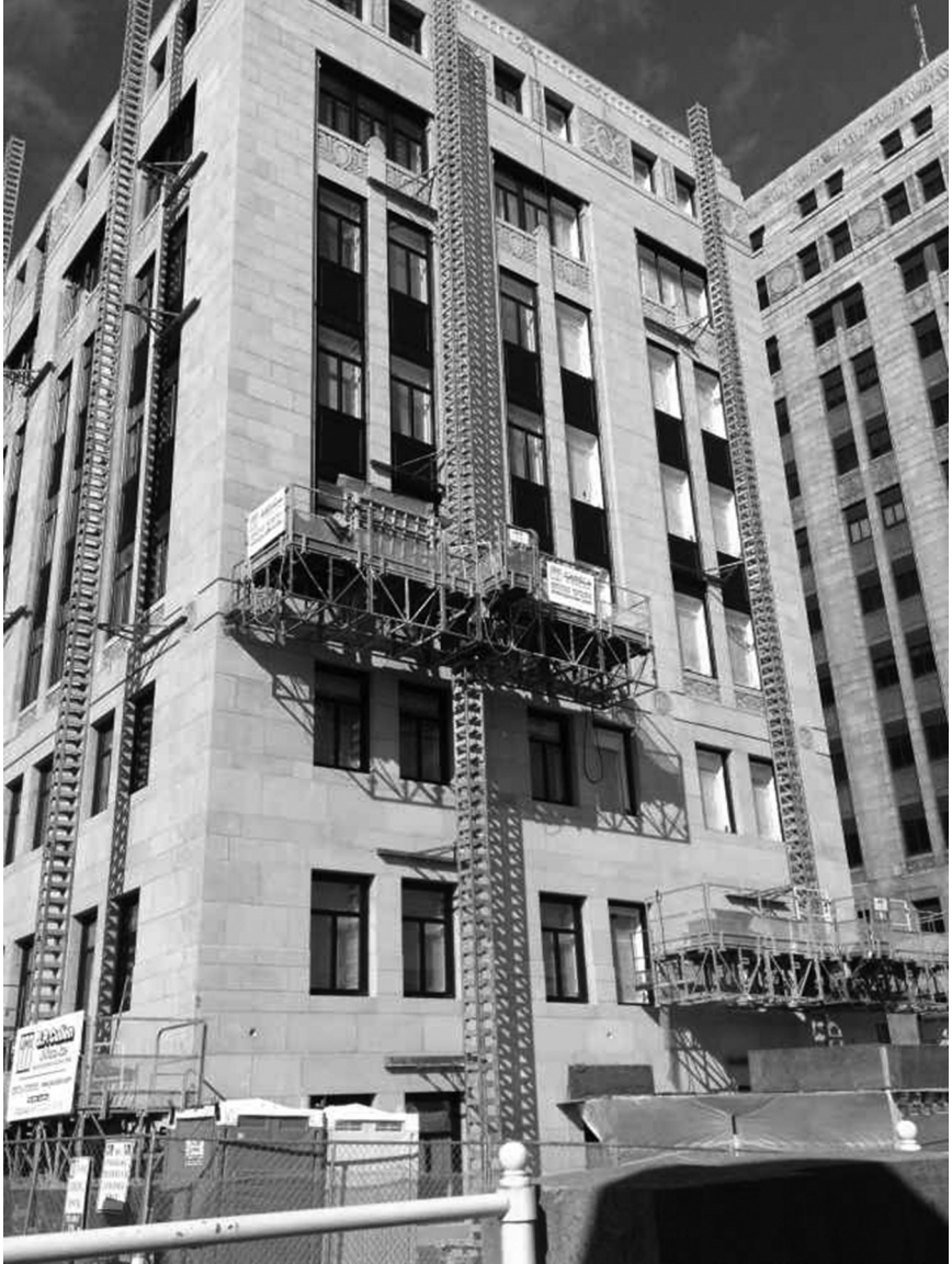
The Department of Health Services building undergoes window replacement in 2013 as part of a $14.5 million, 18-month, restoration project. Construction on the building, which is on the National Register of Historic Places, was begun in 1930, and is built of granite from the State Quarry in Amberg, Wisconsin. (Department of Health Services)
