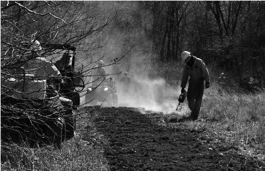
Department of Natural Resources workers test the effectiveness of a fire break prepared around the perimeter of a prescribed burn unit with a test fire. (Department of Natural Resources)
