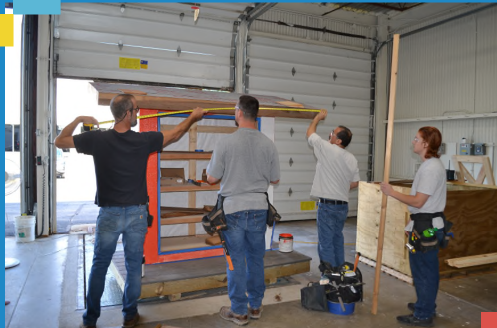
Students working in the Madison College Carpentry Techniques Technical Diploma program
