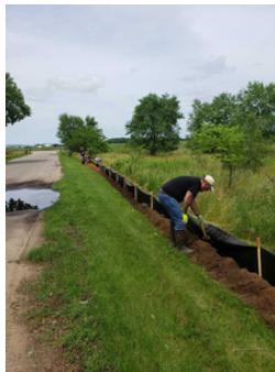
Trench fencing installation. (Nathan Nye)
