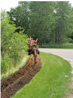
Backfilling a trench. (Nathan Nye)
