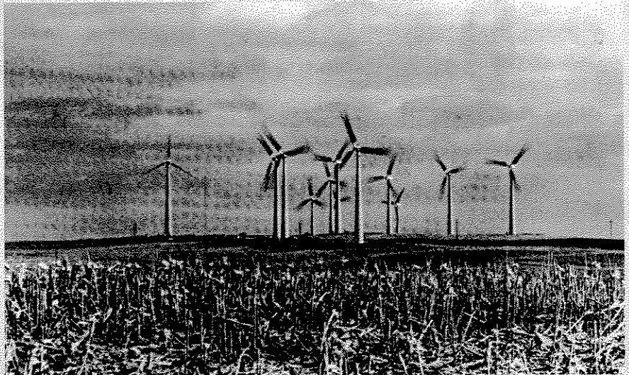
A wind farm in Minnesota.
