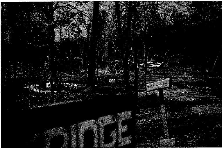
An example of an indefensible property—extinguishing the wildfire that burned this house was virtually impossible because of its close proximity to dense, combustible stands of Ponderosa pine. In addition, drivers of fire protection vehicles found it very difficult to gain easy access to the wildfire because of road conditions and remoteness of the site. Photo: Bill Terry, USDA Forest Service, Northeastern Area.
