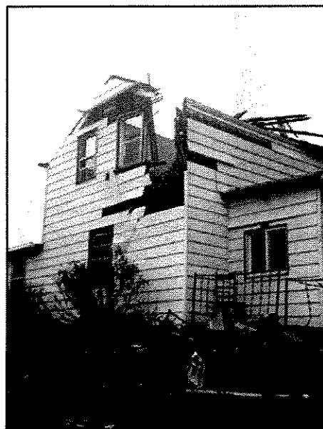
Hail and winds of more than 100 MPH caused damage to many homes and businesses.
