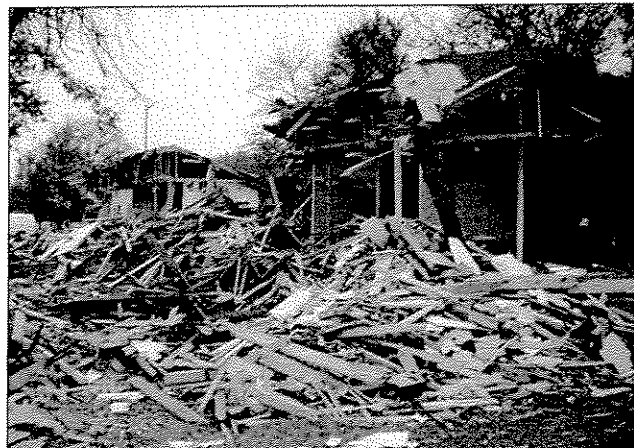
Waste generated at a building demolition project.
