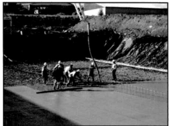
Montagne Farm Swanton, VT Under Construction
