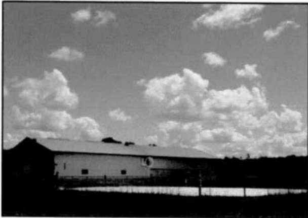
Gordondale Farms Nelsonville, WI 140 kW
