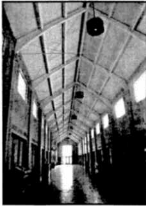
Filter hall at Linnwood Water Treatment Plant
