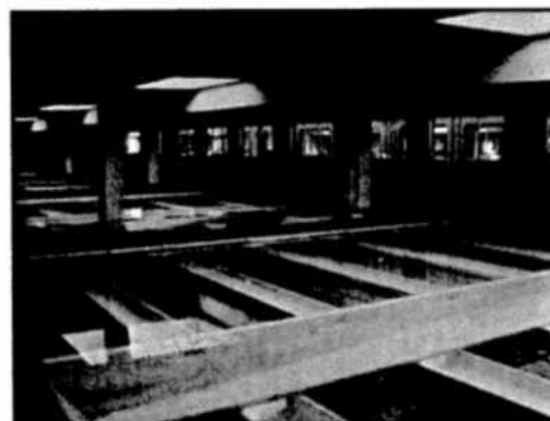
Filter skylights, interior view
