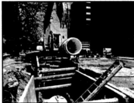
Installation of 36" concrete water main in East Wisconsin Avenue
