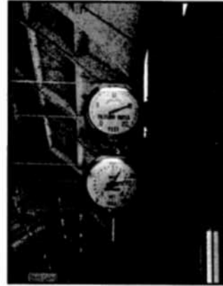
Original 1939 filter gauges no longer in use
