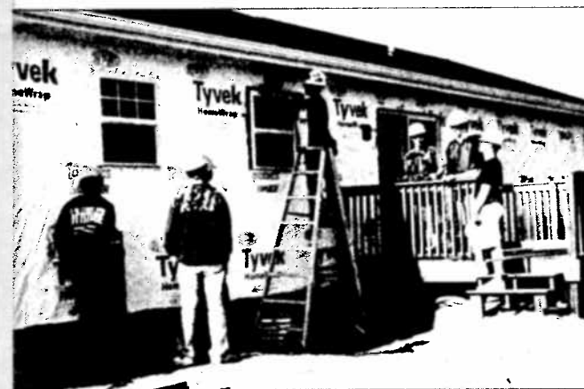
SPASH technology education students work on house #11.
