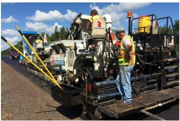
A paving crew working on the WIS 21 enhanced density pilot project demonstrates how density targets may be increased. The idea that higher density leads to improved performance results from the Critical Factors Affecting Asphalt Concrete Durability project.
