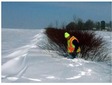
Wind loses speed as it is forced to go around and through the living snow fence, stopping much of blowing snow short of the roadway as it loses the wind's momentum, drops and collects in and around the shrub barrier.
