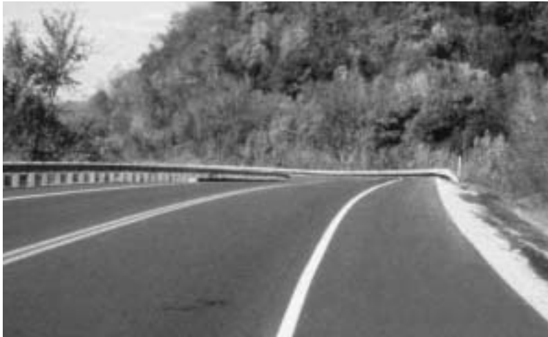
A Typical shoulder Treatment on a rural highway.
