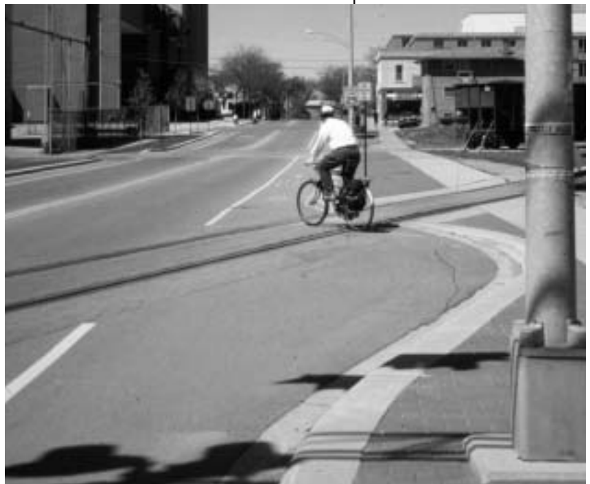
A tapered approach allows bicyclists to cross the railroad tracks at a safe angle.
