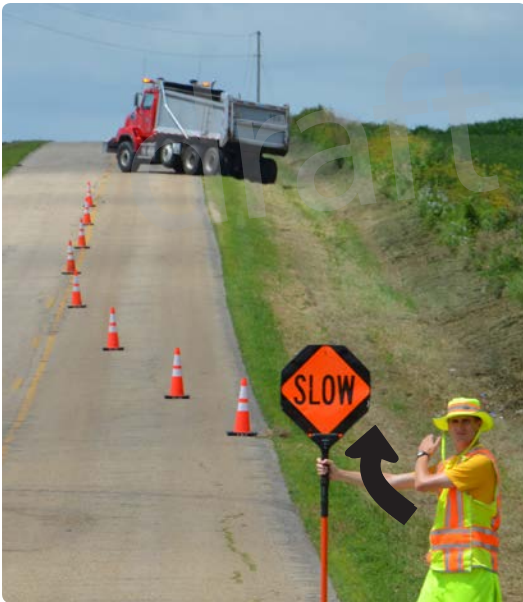
Figure 4: Releasing traffic into the open lane; opposite drive lane
