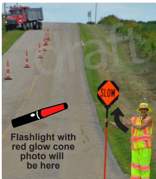
Figure 5: Releasing traffic into the open lane; standard drive lane
