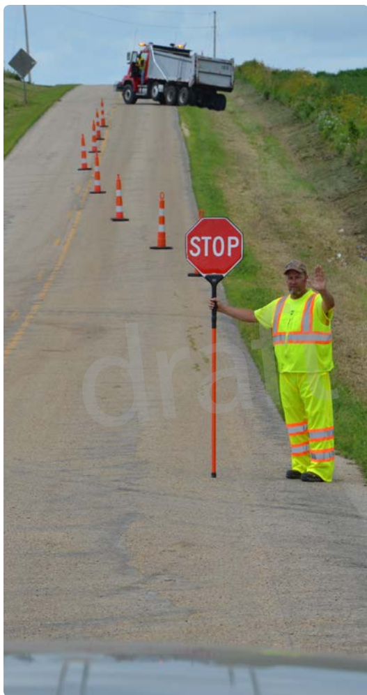
Figure 3: Stopping first vehicle from shoulder
