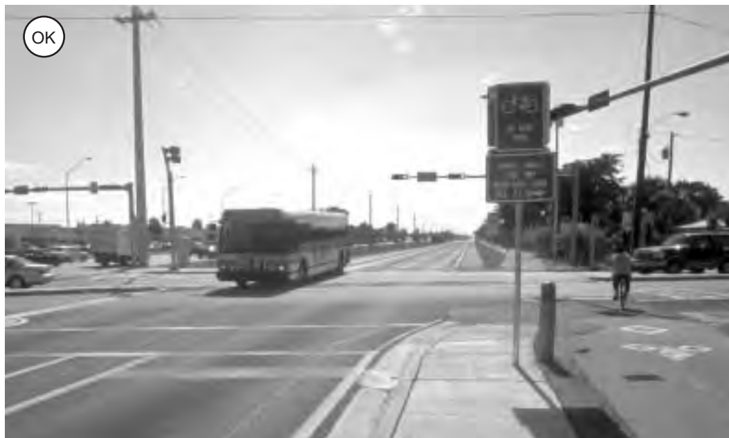
Figure 4-109: This path has few crossings and good visibility at this intersection. Even so, it is important to reduce conflicts between turning and crossing movements. A separate left turn phase for the bus, for example, could help.
