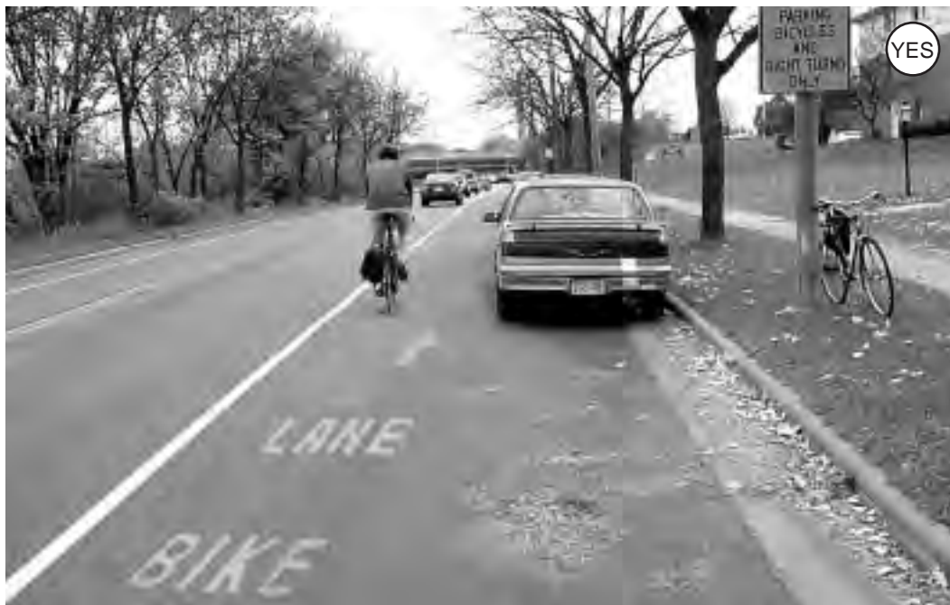
Figure 3-15: Unlike bicycles, motor vehicles are not affected by the joint between the roadway and the gutter pan. As a result, the gutter pan is included when determining the width of the parking lane.
