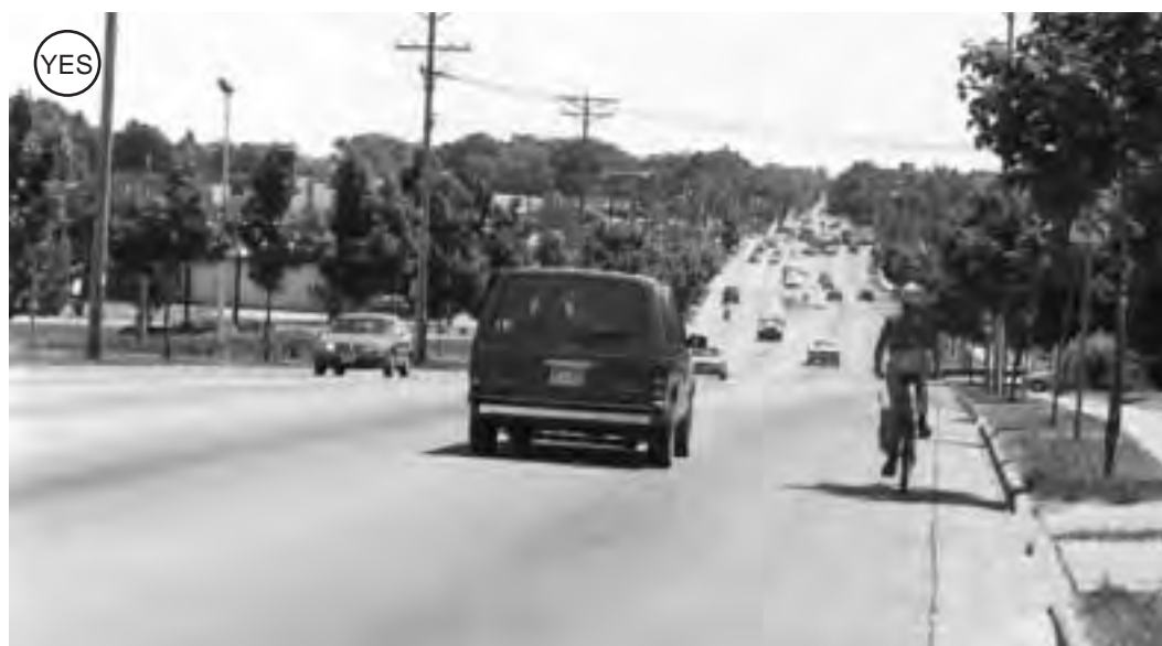
Figure 2-24: A wide outside lane can provide room for bicyclists and motorists to share an arterial or collector street lane.
