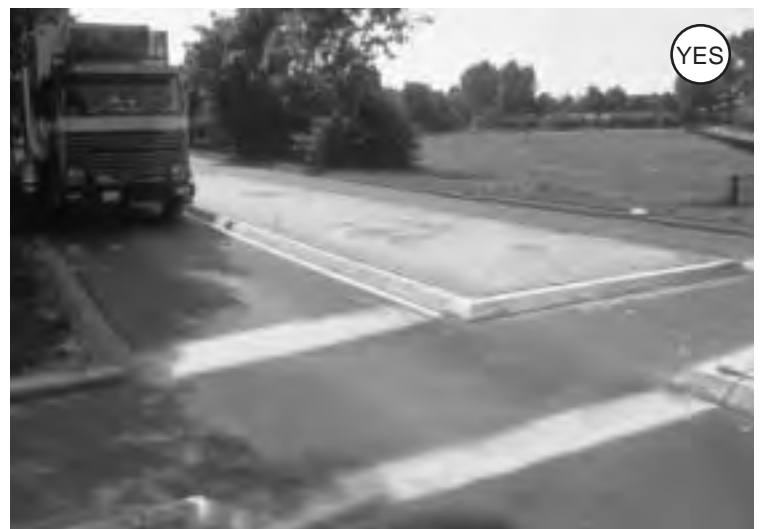
Figure 4-87: A path crossing at a moderate volume highway combines a raised median refuge with signing and marking.
