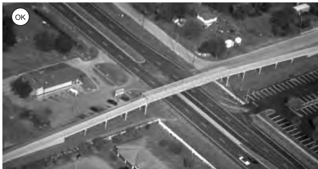
Figure 4-114: Overpass approach ramps are typically longer than ramps for underpasses and can significantly increase costs.
