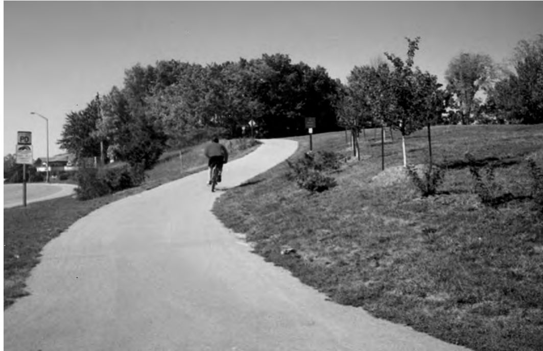
Figure 4-27: Shared-use paths should be designed for all ages. Grades should be carefully considered and should be safe for kids riding coaster brake bicycles.
