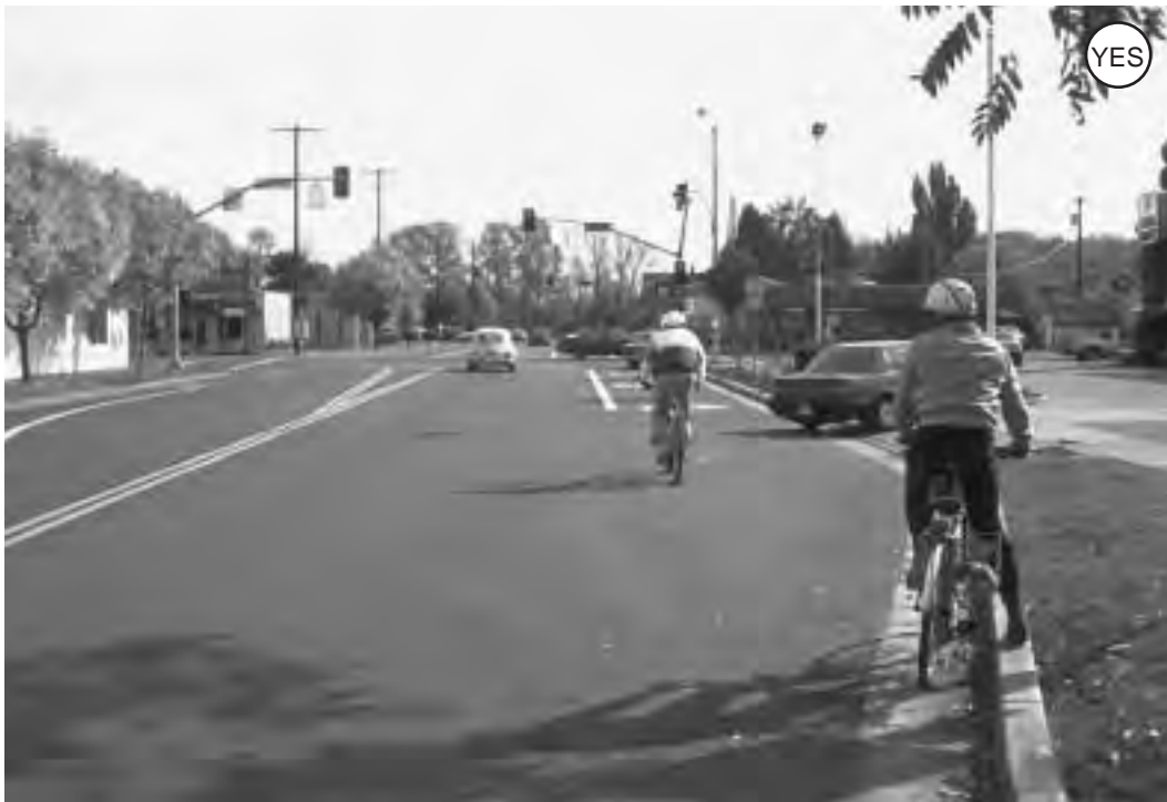
Figure 2-60: At the end of a bridge with wide outside lanes, the extra width should continue in the through lane rather than the right turn lane.
