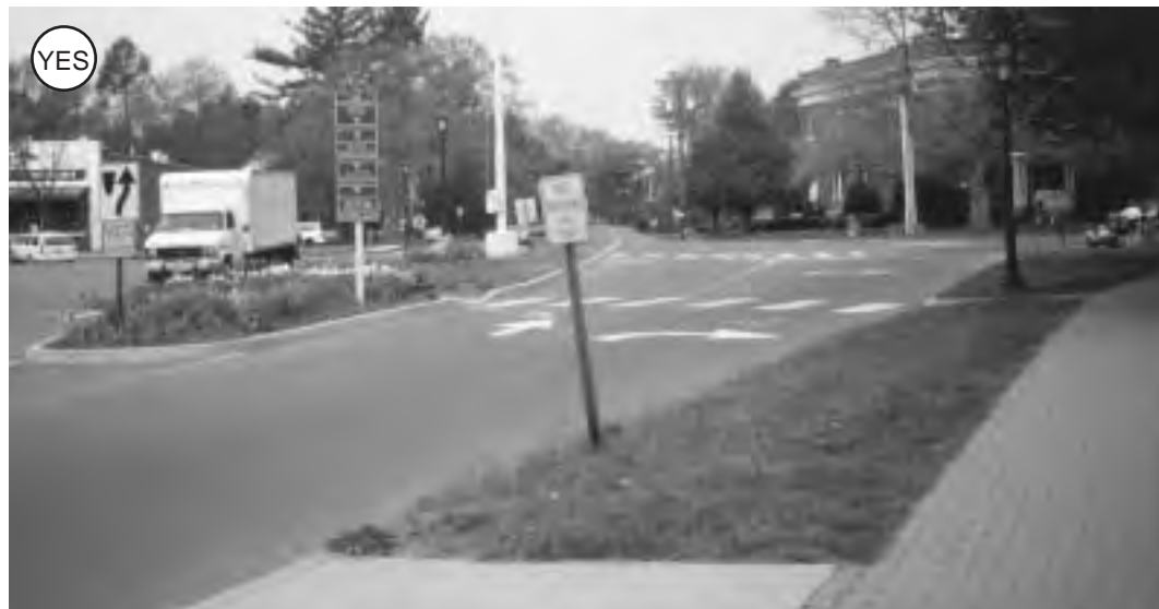
Figure 2-70: A raised median stops motor vehicle cross traffic and left turns. Curb ramps and cuts provide bicycle and pedestrian access.
