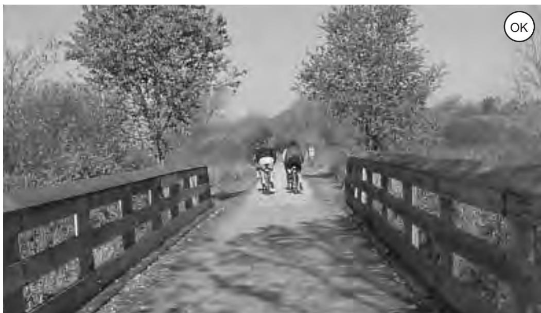
Figure 4-19: A popular unpaved shared-use path following an abandoned railroad line.
