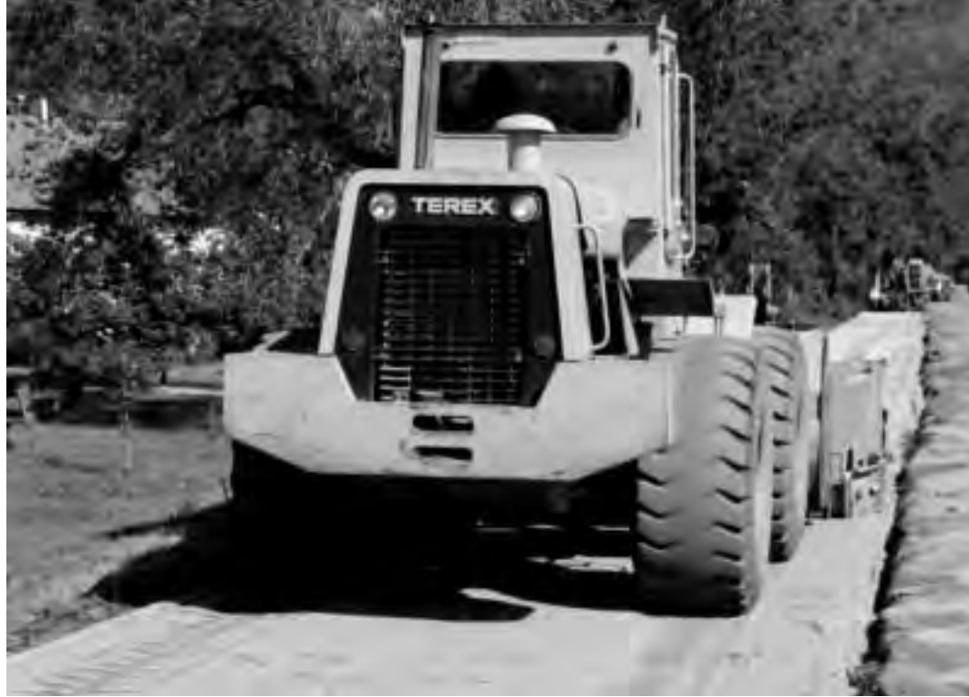
Figure 4-41: Preparing shared- use path subgrade.
