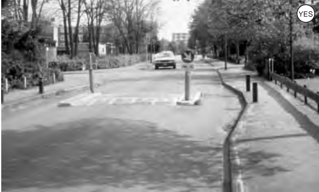
Figure 2-78: A squeeze point with a speed hump narrows motor vehicles lanes but includes bicycle bypasses to the outside. This example also includes a speed hump. As with any traffic calming measure, they must be designed to work with maintenance and emergency vehicles.
