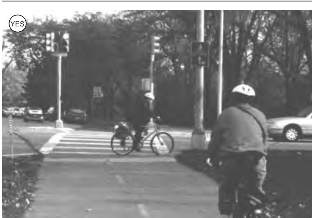
Figure 4-106: An urban crossing that takes advantage of an adjacent signalized intersection. A bicycle signal loop detects bikes to change the signal. Note high-visibility crosswalk marking.
