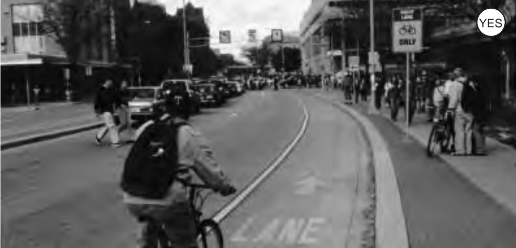
Figure 3-23: The three primary elements that identify a bicycle lane: regulatory signs, lane striping, and pavement markings.
