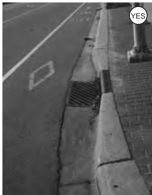
Figure 2-17 (left): Locate drainage grates before the crosswalks and corners to reduce the hazards for wheelchair users and bicyclists.
