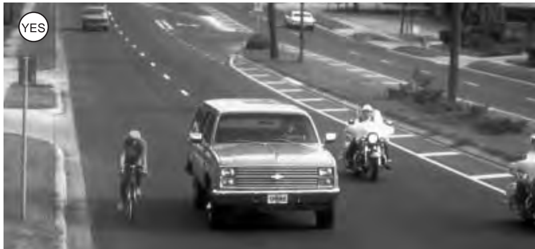
Figure 2-29: One way to gain extra width in the outside lane is to shift the lane striping after a pavement overlay.
