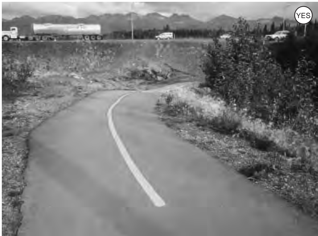
Figure: 4-26: An example of centerline striping used in a curve to separate bicyclists going opposite directions. In this case, no curve widening was used, however vegetation has been trimmed back to improve sight lines.
