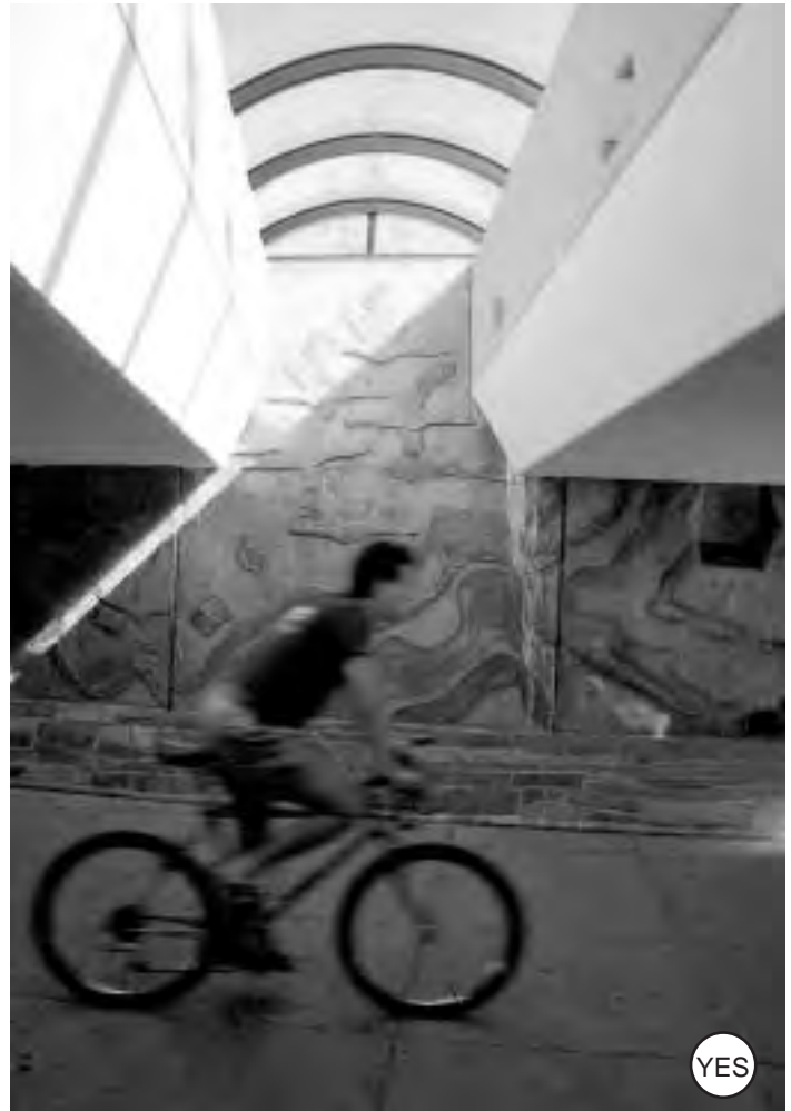
Figure 4-128: This skylight, which comes up into the roadway median above, makes the underpass more inviting.
