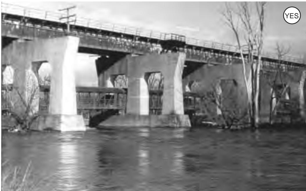
Figure 4-130: This path bridge spans a river under a railroad bridge. Attention must be paid to flood water levels and the river's navigability.
