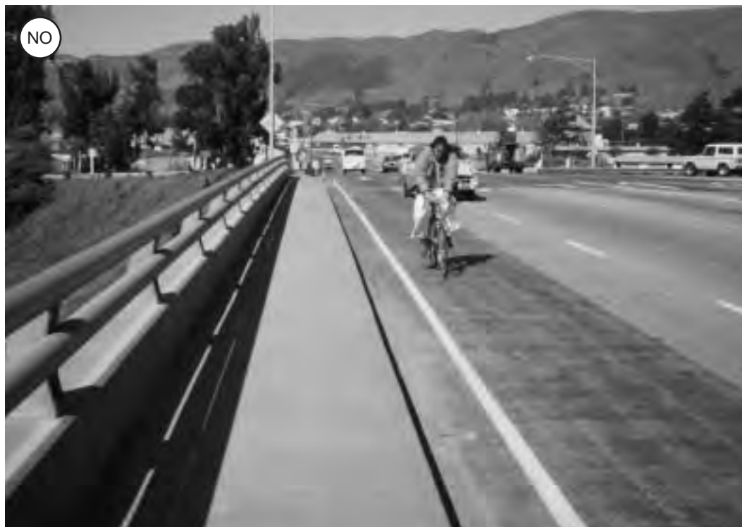
Figure 2-59: On this bridge, debris collects in the narrow striped shoulder; as a result of the surface conditions and the shoulder's width, motorists must change lanes to pass safely.
