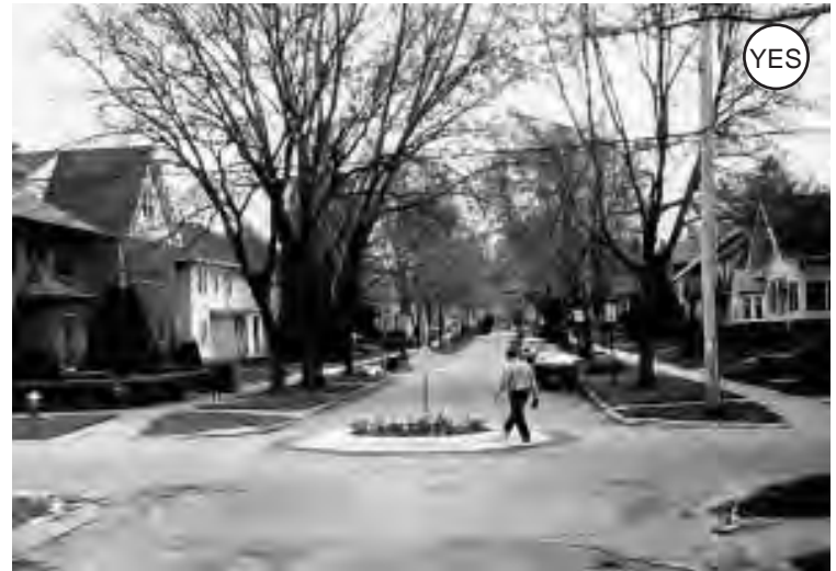
Figure 2-4: Residential streets may require traffic calming measures like this traffic circle. However, designs should not endanger or discourage bicyclists.
