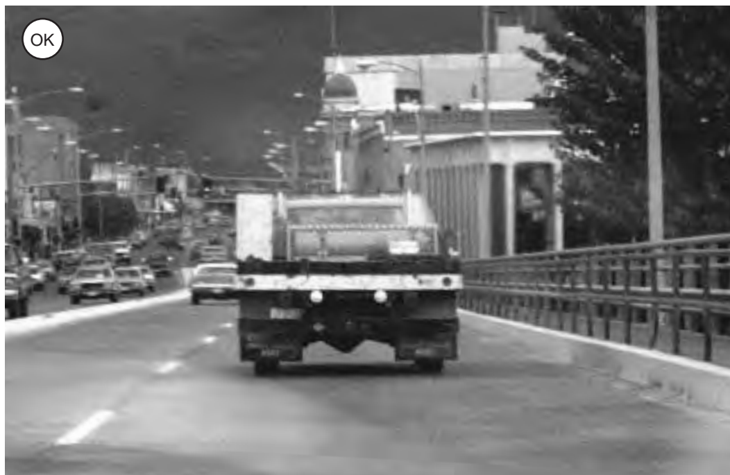
Figure 2-54: Lane striping was shifted to the left on this 4-lane downtown bridge to give 15-foot outside lanes and 11-ft. inside lanes.
