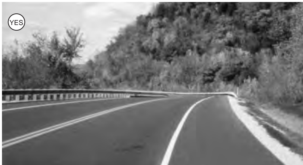
Figure 2-8: Basic paved shoulders are often the only improvements needed to make rural roads more bicycle-friendly.
