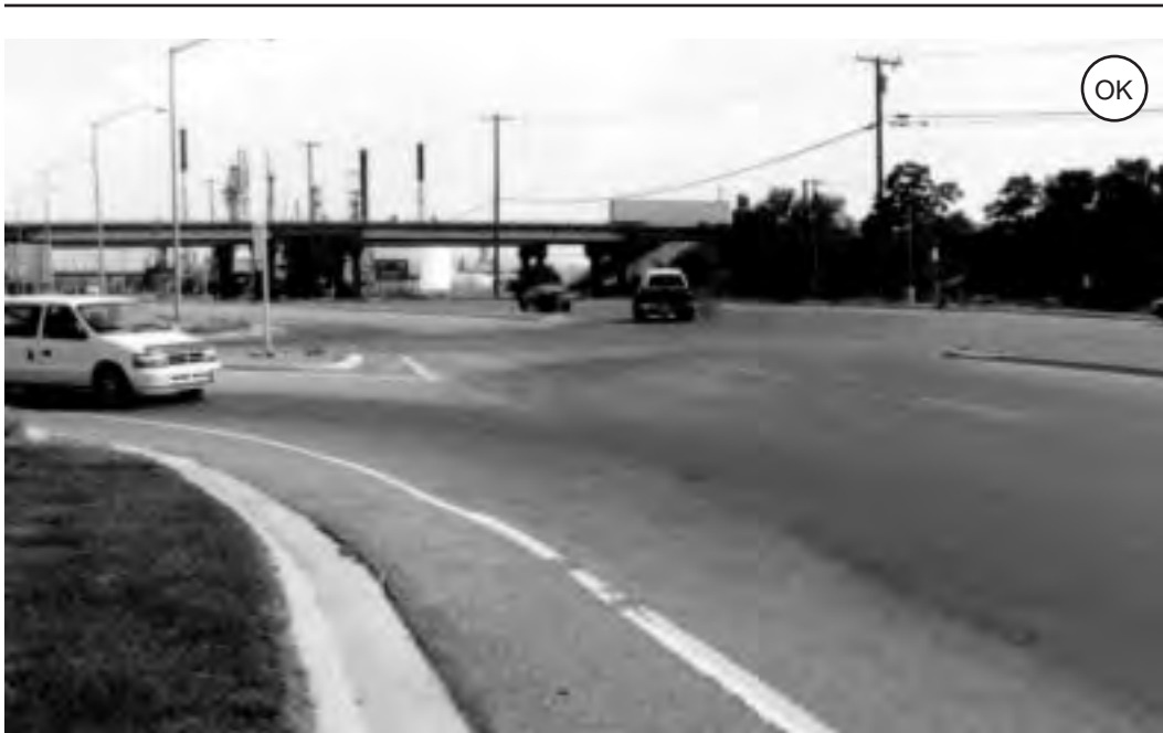
Figure 2-63: An interchange appropriate for a rural location but not a suburban or developing area.
