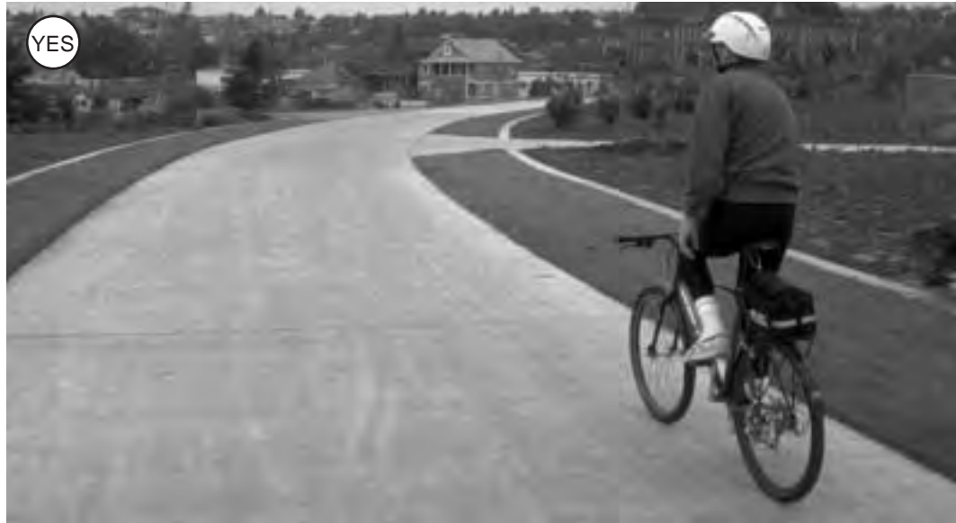
Figure 4-44: Concrete can provide a smooth and long-lived surface, as shown on this shared-use path.
