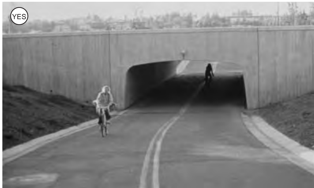
Figure 4-127: With good sight distances and visibility through to the other side, this structure provides a comfortable passage for bicyclists.
