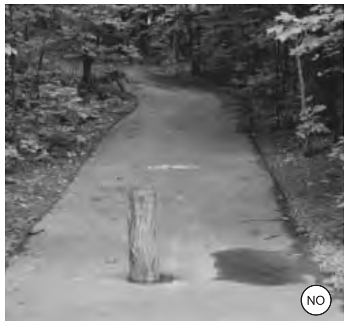
Figure 4-153: Natural wood posts in unlit areas are hard to see.
