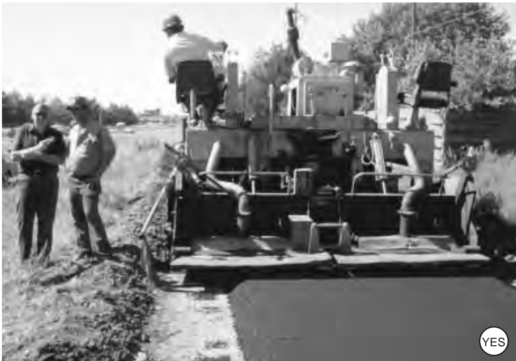
Figure 4-42: Machine-laid asphalt is smooth and a common surface for shared-use paths.
