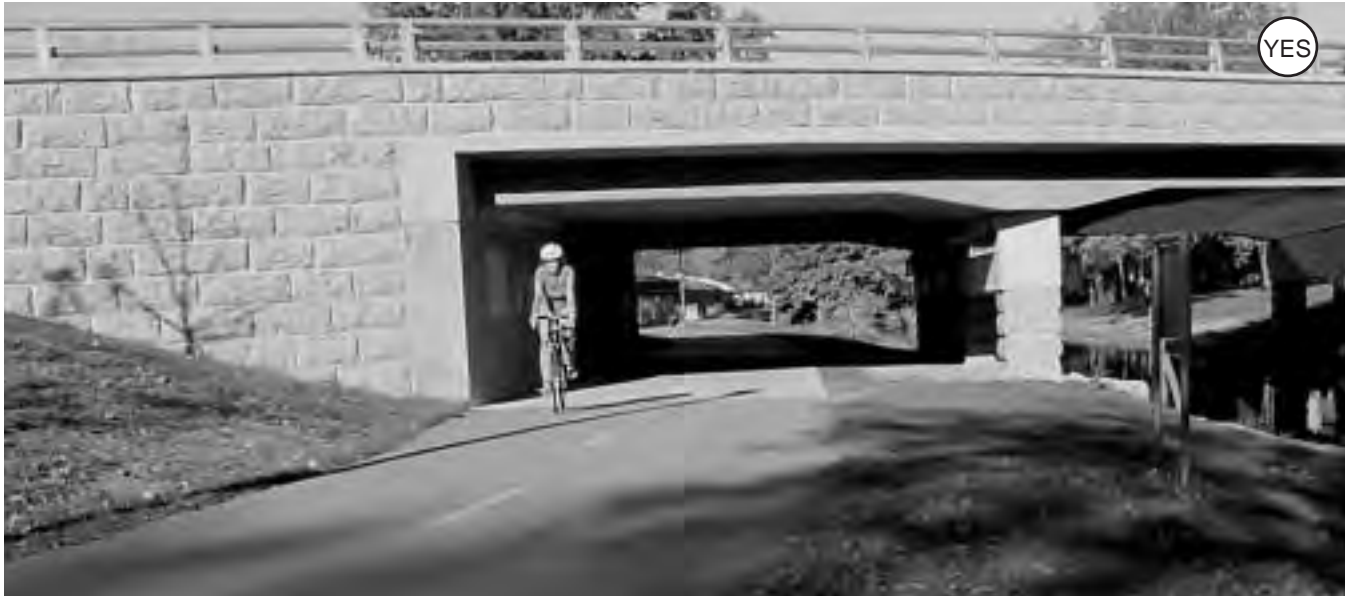
Figure 4-125: Careful design can result in an open underpass that is inviting to users.
