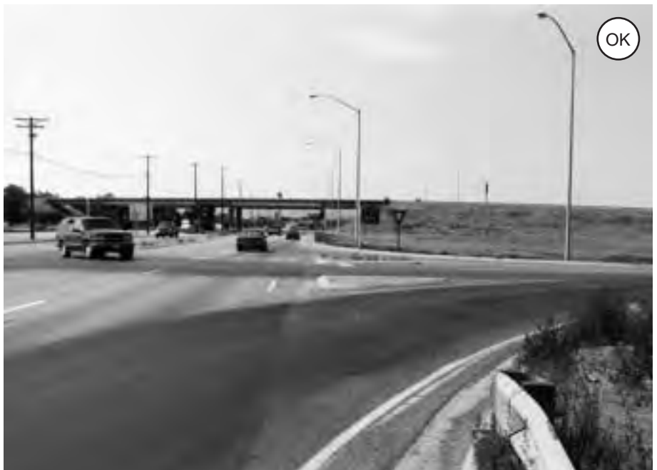
Figure 3-45: Interchanges with high-speed turns and merges are suited only to an environment that will remain rural.
