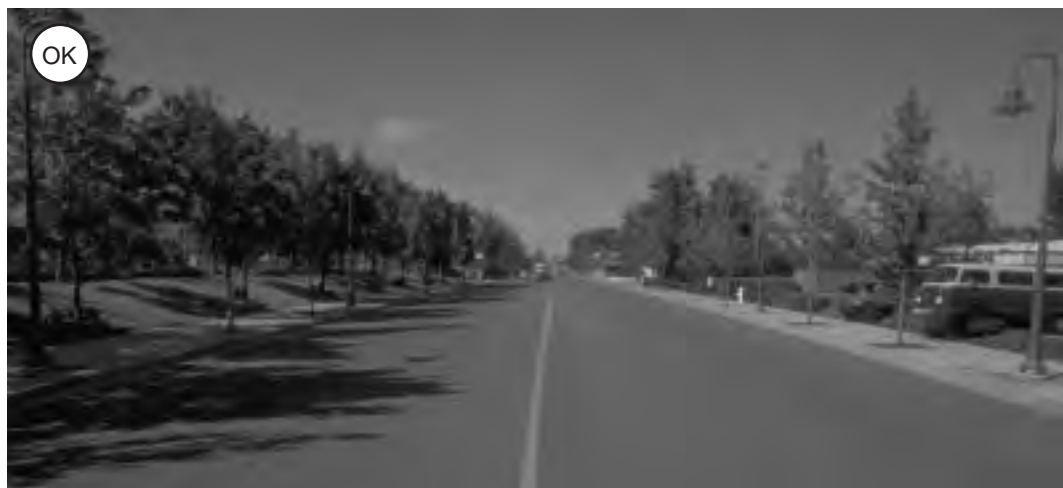
Figure 2-5: In some areas with plenty of off-street parking, collectors are designed for on-street parking with extra space for bicycles. This may result in excessive width and potentially high traffic speeds.
