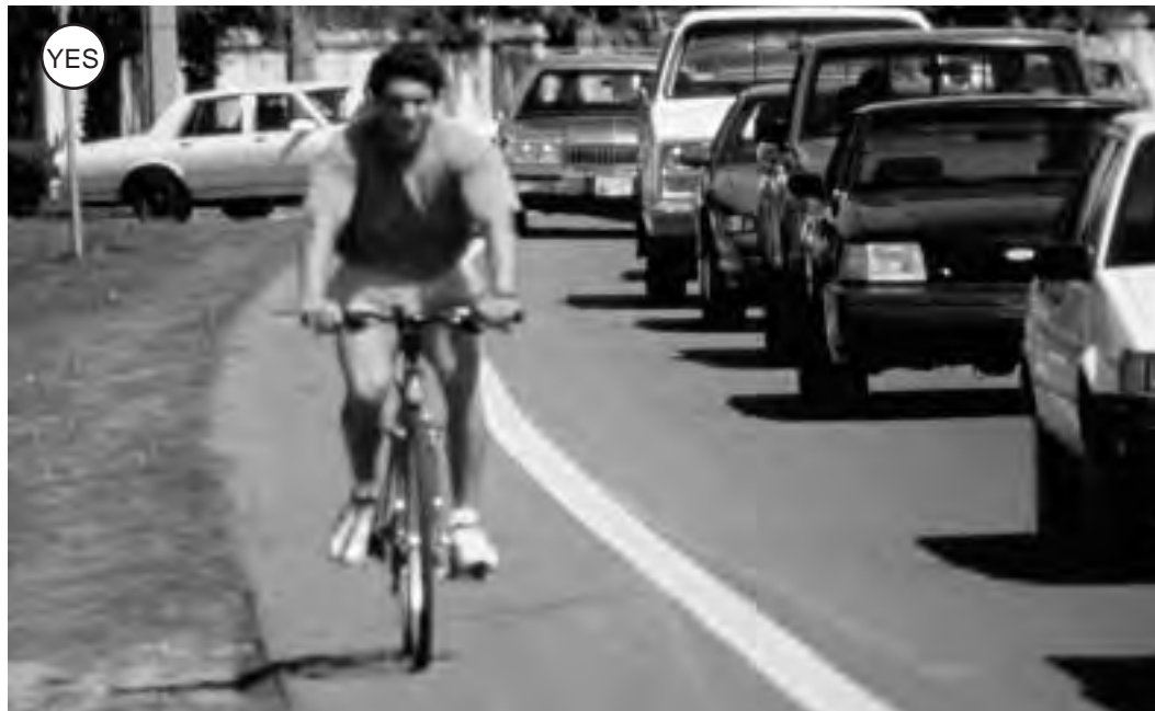
Figure 3-20: Striping bicycle lanes on roadways without curbs can be an important improvement in fast growing suburban and exurban areas.
