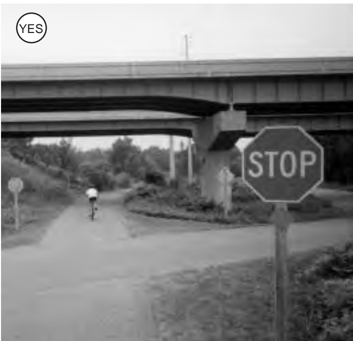
Fig. 4-81: A shared-use path follows a river corridor and takes full advantage of a grade separation with a freeway.
