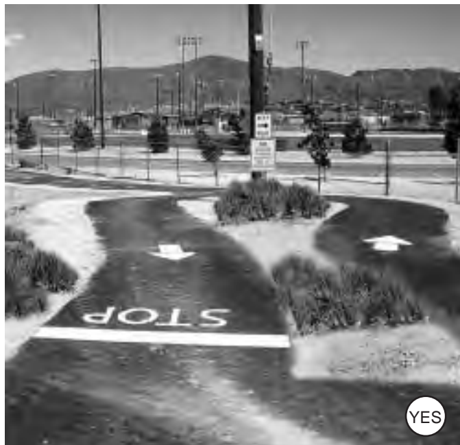
Figure 4-149: A split path entrance can, with proper low plantings, discourage motorists from entering.
