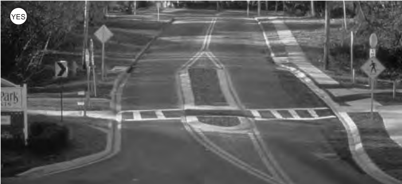
Figure 4-99: Traffic calming measures can make a significant difference in how easily path users can get across a roadway.
