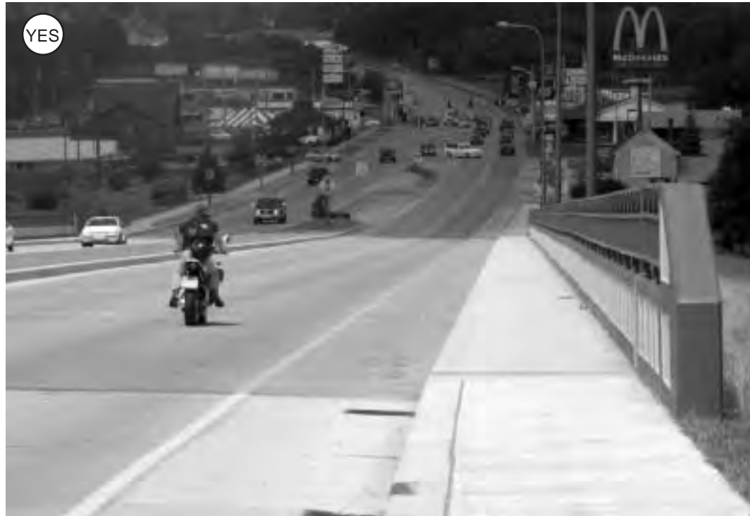
Figure 2-55: A suburban bridge with 5-ft shoulder for bicycles, as well as a sidewalk.
