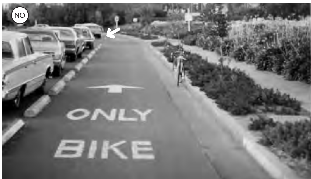
Fig. 3-5: A bicycle lane to the right of parked cars creates sight obstructions, keeping bicyclists and turning or crossing motorists from seeing each other. This is particularly dangerous at intersections and driveways (see arrow). In addition, crossing pedestrians may not notice – or be noticed by – bicyclists.
