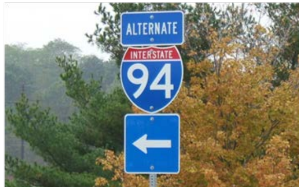
Figure 13.1 - Emergency Alternate Route Signing
