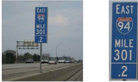
Figure 5.1 - Enhanced Reference Marker Example: I-94 EB at Mile Marker 301.2
