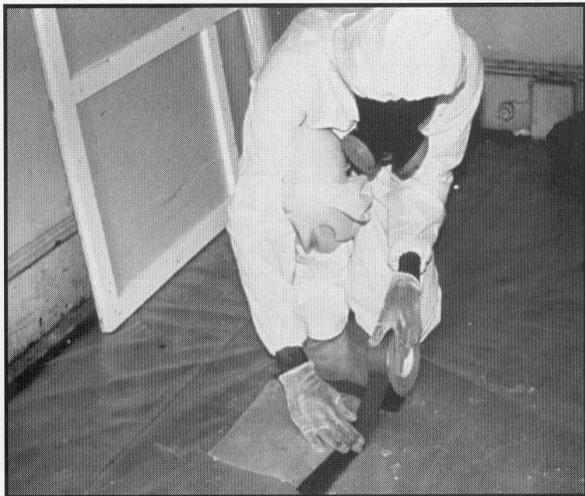
Figure 14.7 Plastic Sheeting Should Be Repaired as Part of Daily Cleanup.
