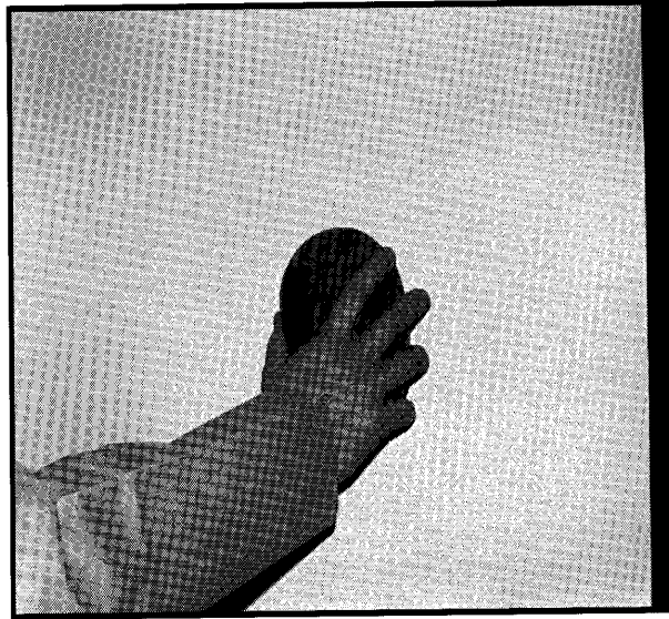
Figure 11.4 Use a Sponge To Wet Sand and Smooth New Patching Material.
