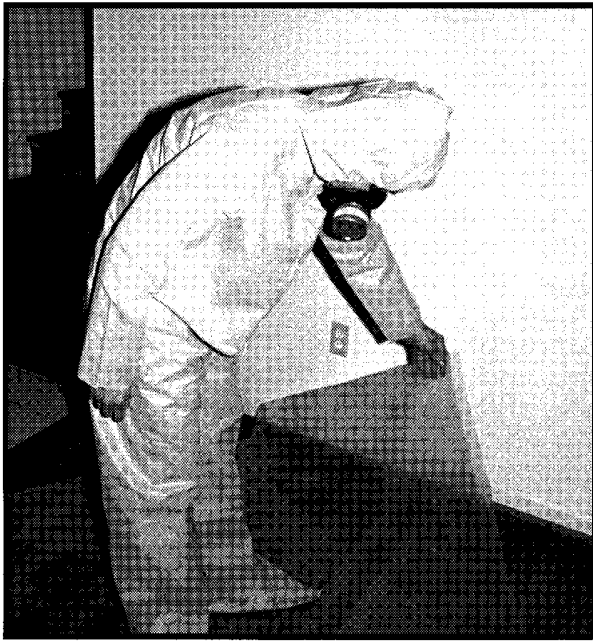
Figure 14.8a Pick Up Corners of Plastic Sheeting.
