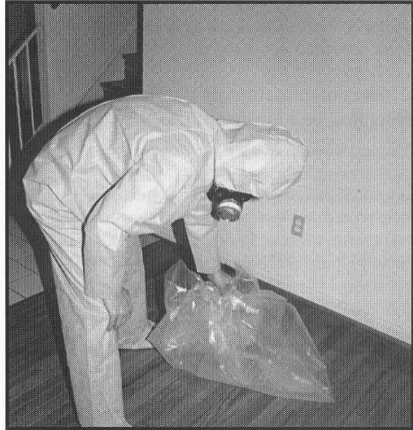
Figure 14.8b Fold Plastic Inward.
