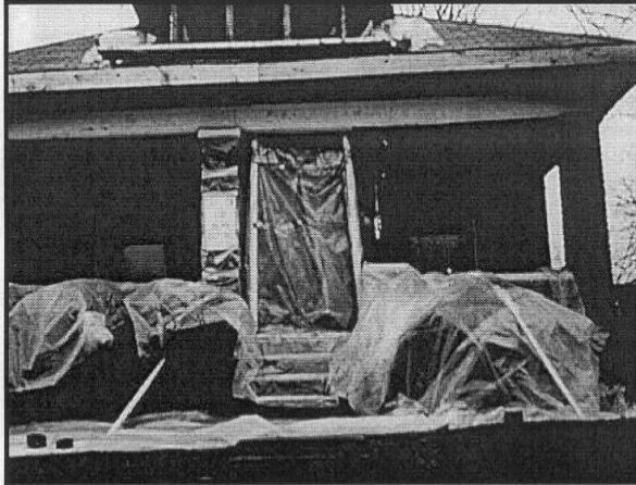
Figure 8.3b Prepare the Worksite With Plastic Sheeting (exterior).
