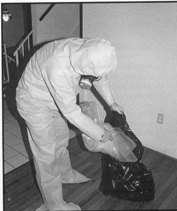
Figure 14.8c Dispose of Plastic Sheeting in a Plastic Trash Bag.
