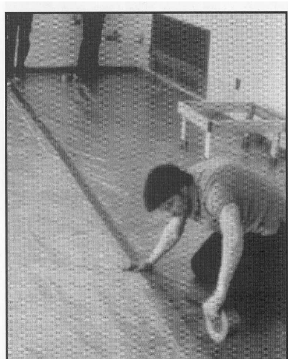
Figure 8.3a Prepare the Worksite With Plastic Sheeting (interior).
