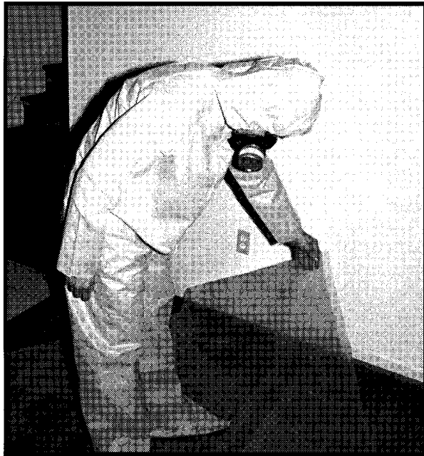
Figure 14.8a Pick Up Corners of Plastic Sheeting.
