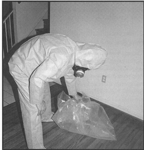
Figure 14.8b Fold Plastic Inward.
