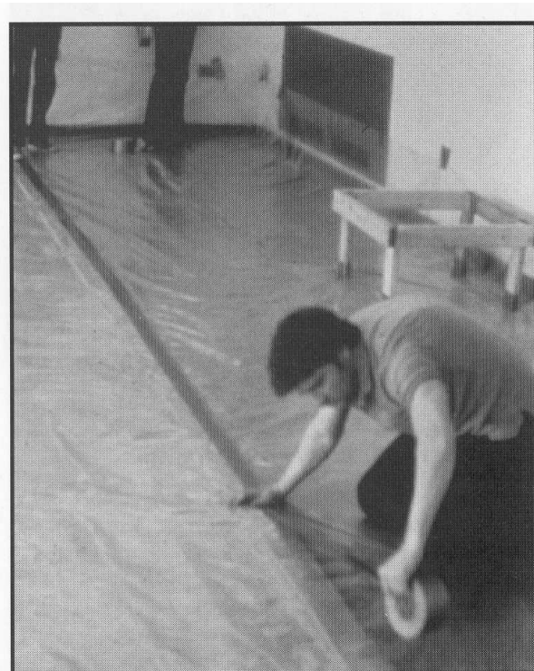
Figure 8.3a Prepare the Worksite With Plastic Sheeting (interior).
