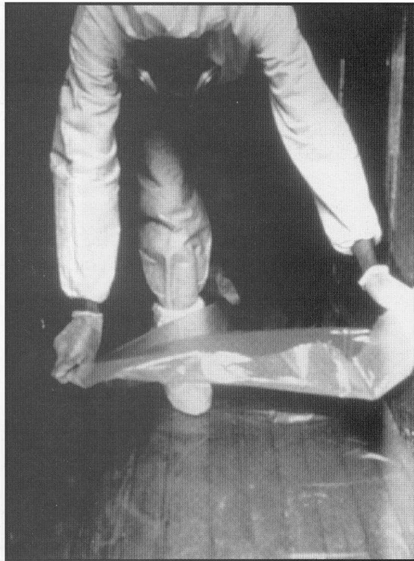
Figure 8.4 Apply a Second Layer of Plastic.
