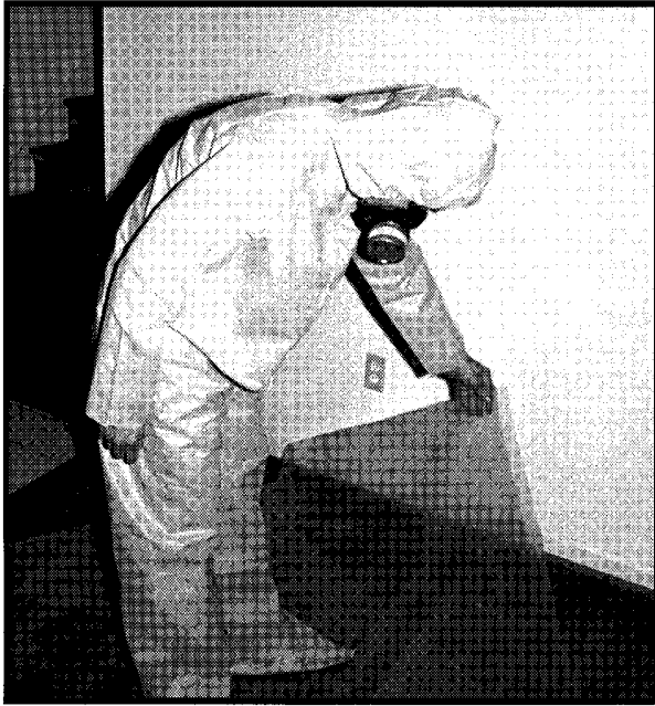
Figure 14.8a Pick Up Corners of Plastic Sheeting.
