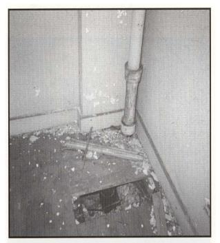
Figure 14.6 Precleaning Is Needed in Areas Where Contamination and Deterioration Are High.
