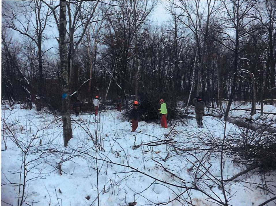
Figure 3. Brush is piled for rabbit habitat, for burning, or to be bundled for river channel placement.
