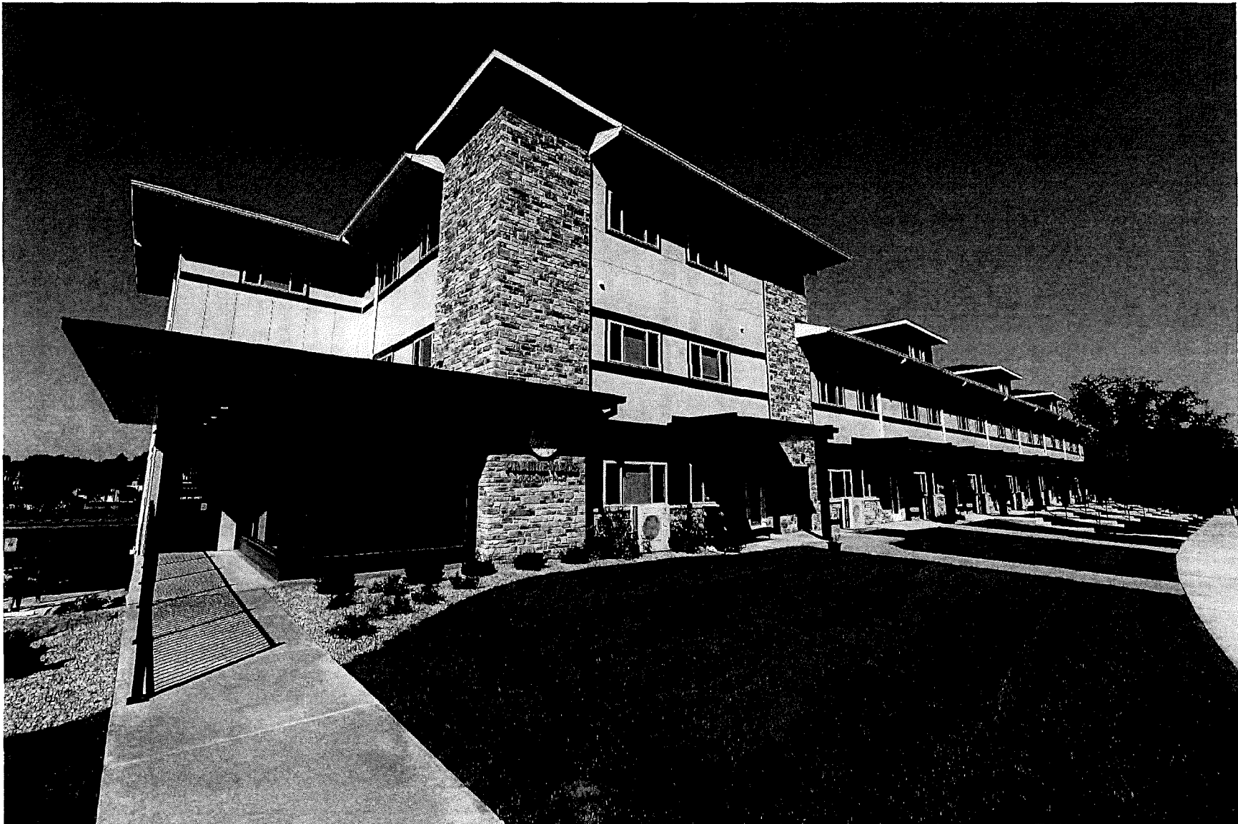
Prairie Haus – 30 workforce housing units and 10 units for adults with disabilities in New Glarus Wisconsin Housing Preservation Corp
