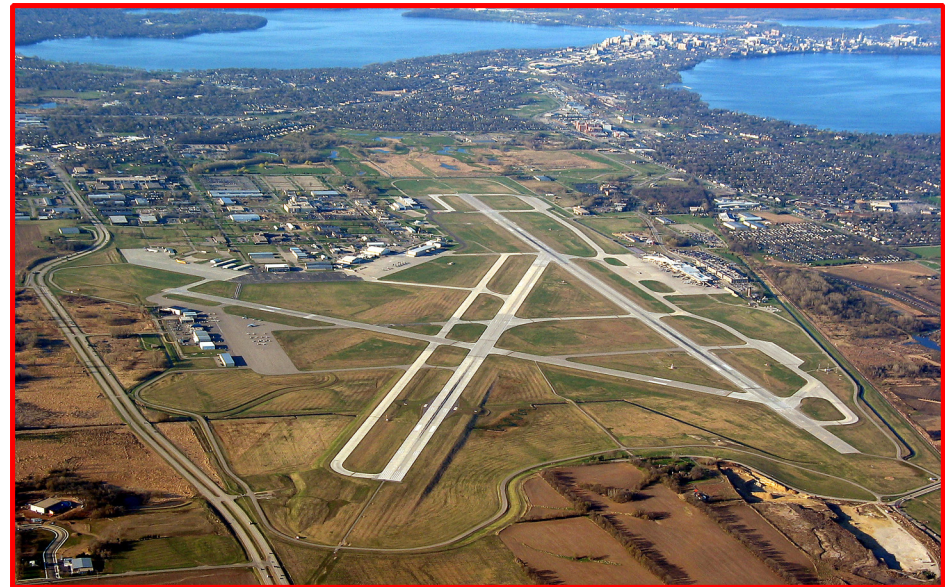
Dane County Regional Airport (MSN)
