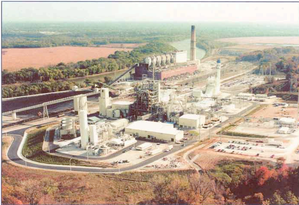
The Wabash River Coal Gasification Repowering Project
