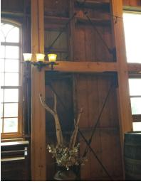
7 trusses for support for snow and wind load
