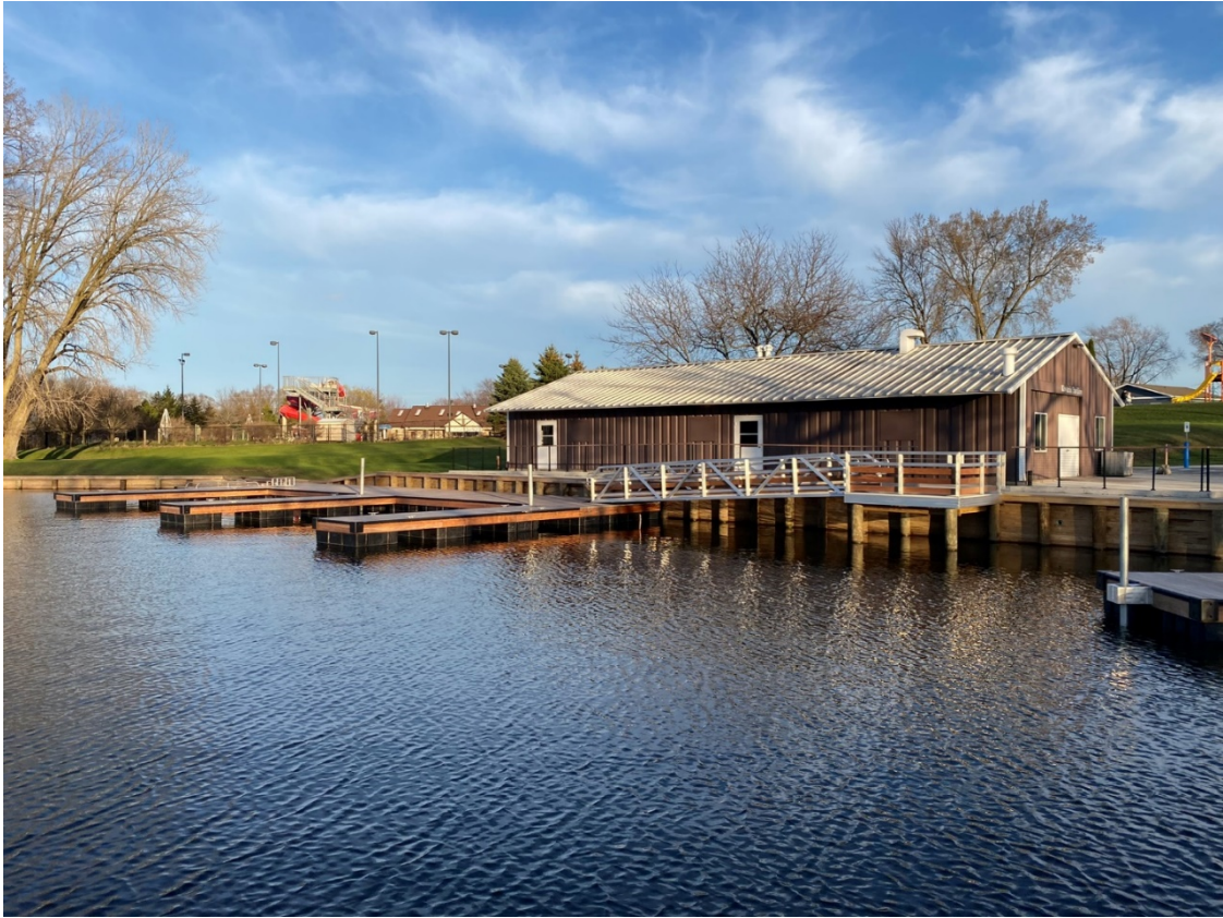
New Transient Boating Floating Pier, Seawalls, and Canoe/Kayak Launch
