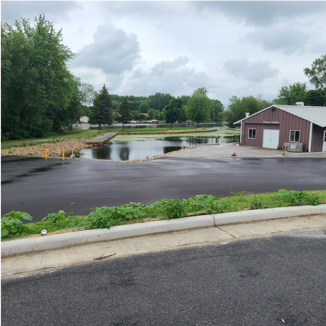
Reconstructed Boat Launch, seawalls, and ADA Parking
