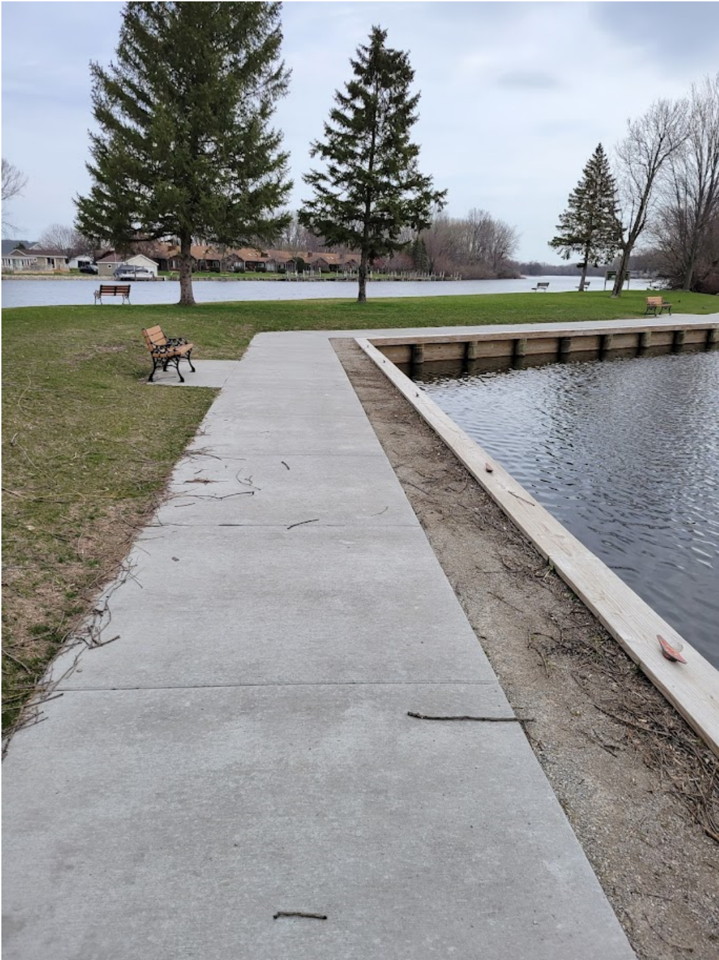
New Seawalls and ADA Sidewalk
