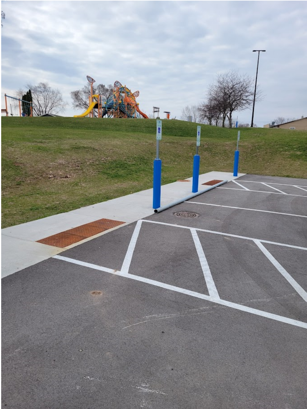
New Boat Ramp ADA Parking
