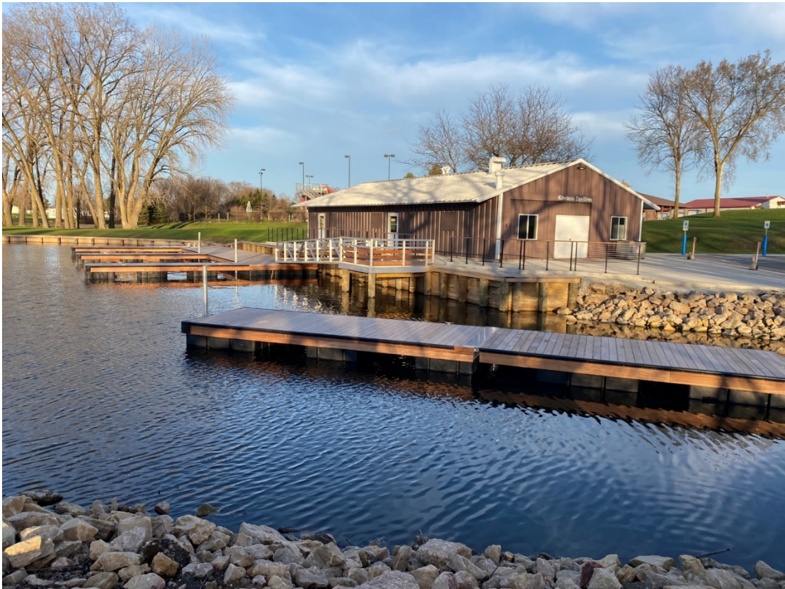
New Transient Boating Floating Pier, New boat Ramp and Pier
