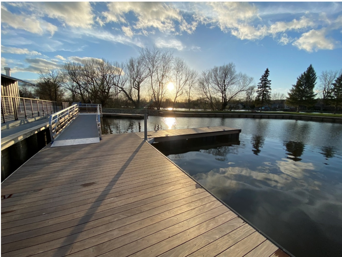
New Transient Floating Boating Pier
