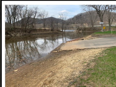
Existing launch panels, note orientation and asphalt approach
