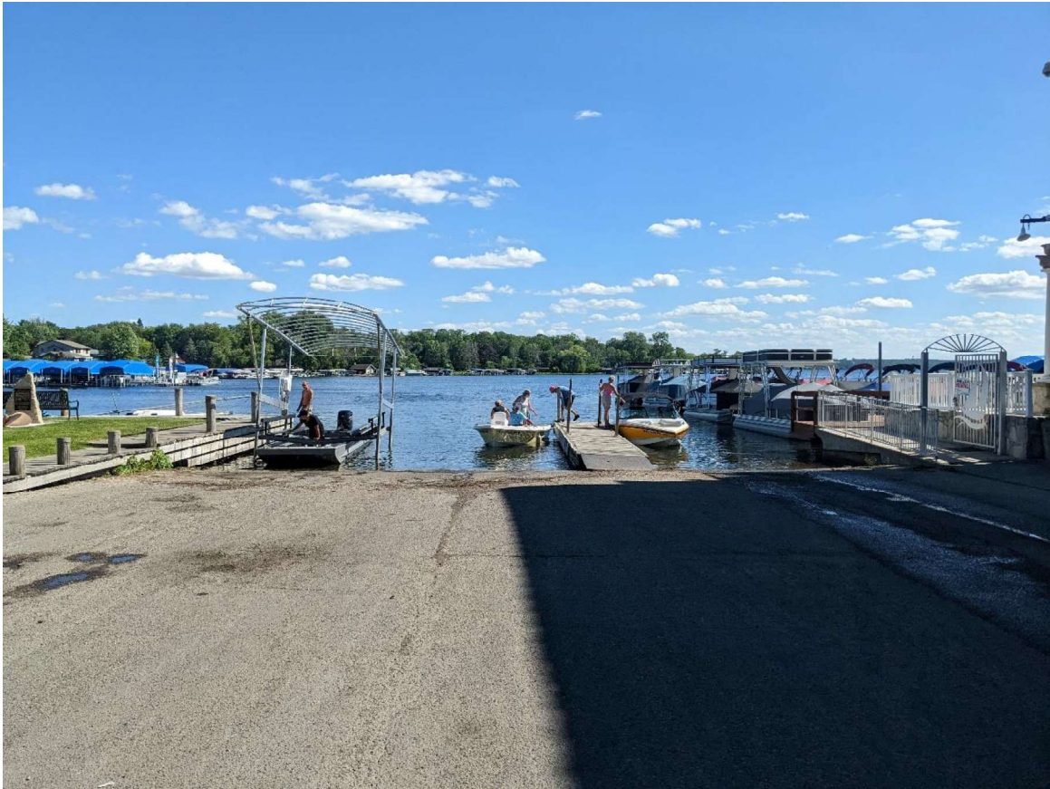
Existing boat launch and non-ADA compliant boarding dock that is offset on the launch, causing confusion and congestion.
