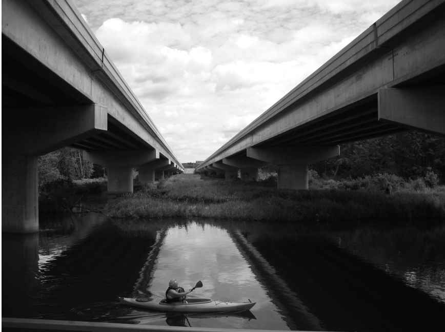
A kayaker paddles under newly constructed U.S. Highway 10 bridges spanning the Wisconsin River near Stevens Point. (Department of Transportation)
