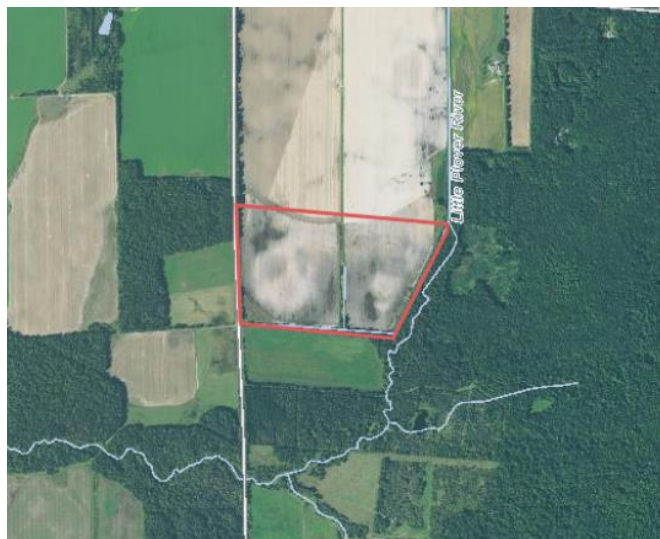
The Plover Soik ILF project is located in Portage County in the Village of Plover, next to the headwaters of the Little Plover River.
