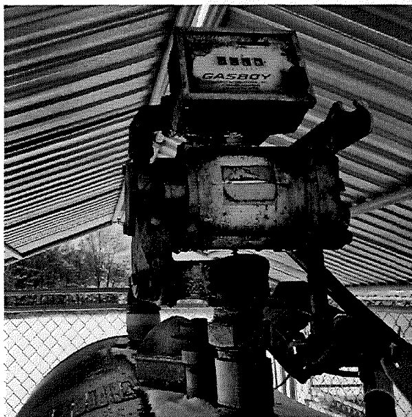
Neglected leaking from pump
